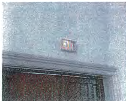
Incandescent Exit Light, One Lamp Out
