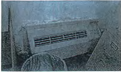
Thru-wall Mechanical unit
