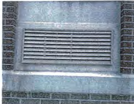
Exterior Through Wall Unit Louver
